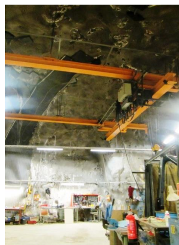
The underground workshop
