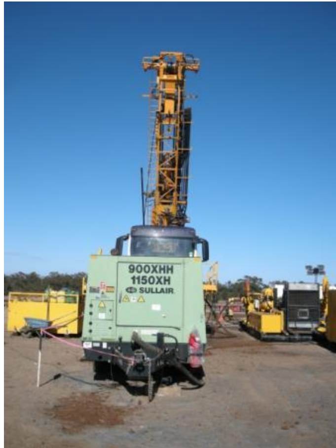
Figure A.16: An example of an air compressor set up at the rig drilling an open/chip borehole
