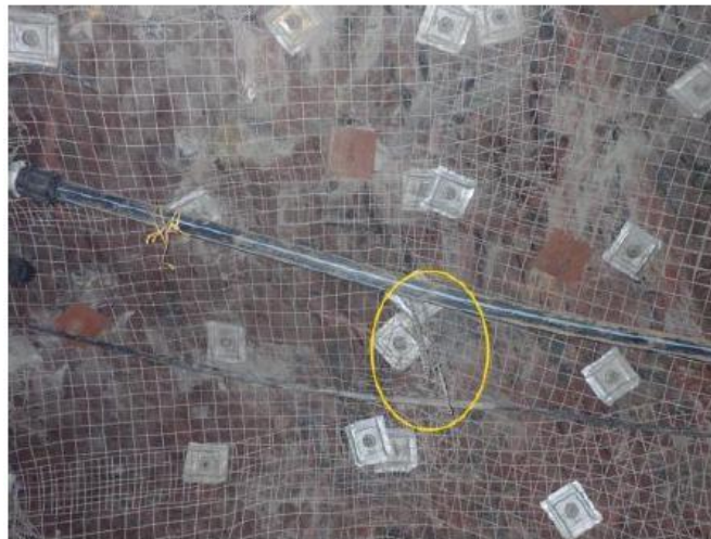
View of the failed chain installed to secure the air line to the backs.
