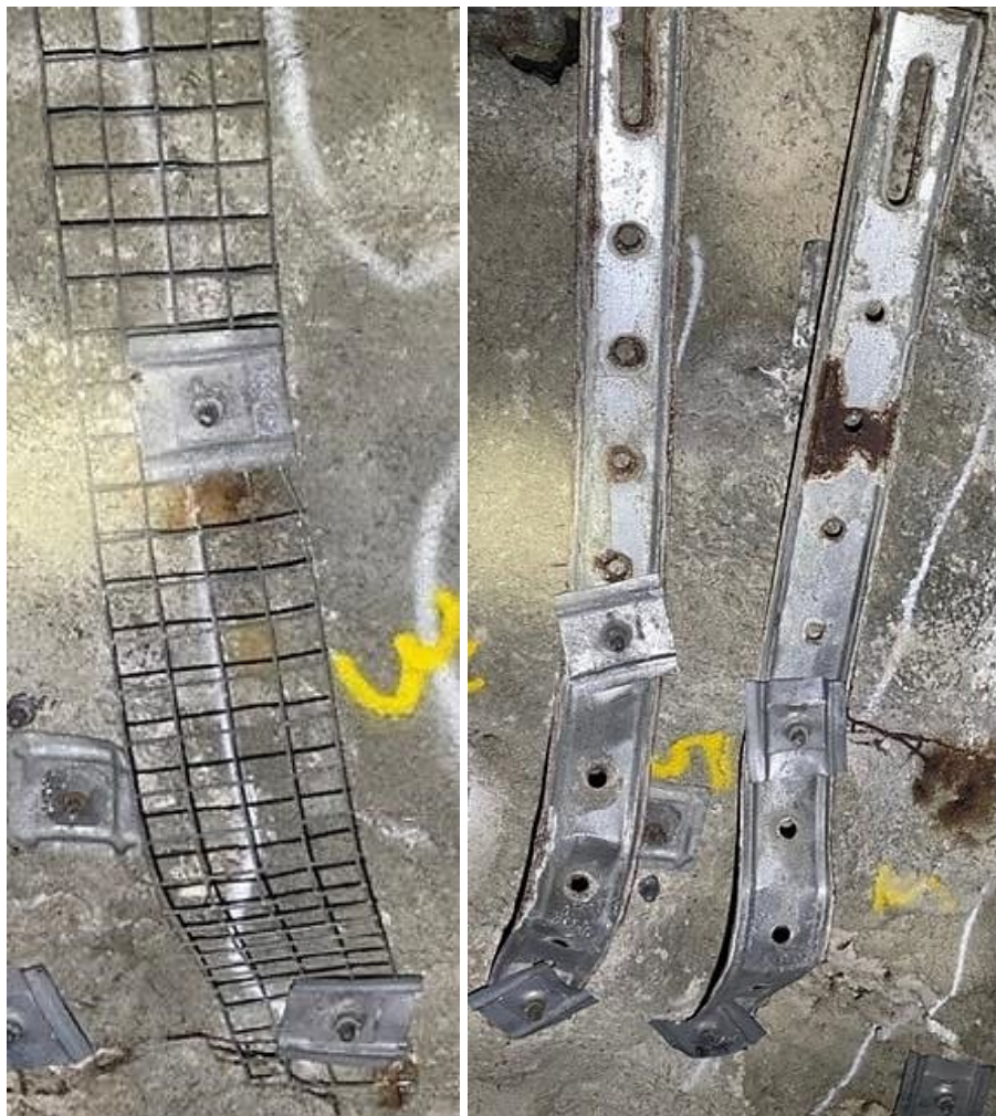
FIG 1 – (left) Installed Mesh strap; (right) W-straps.
