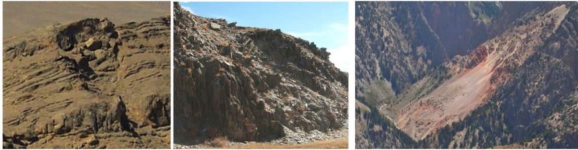
FIG 4 – Slope failures belonging to Category II involving combined shearing and sliding or flexural toppling.
