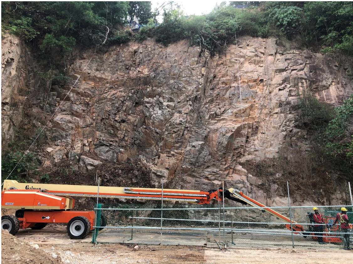
FIG 2 – The old quarry wall slope.
