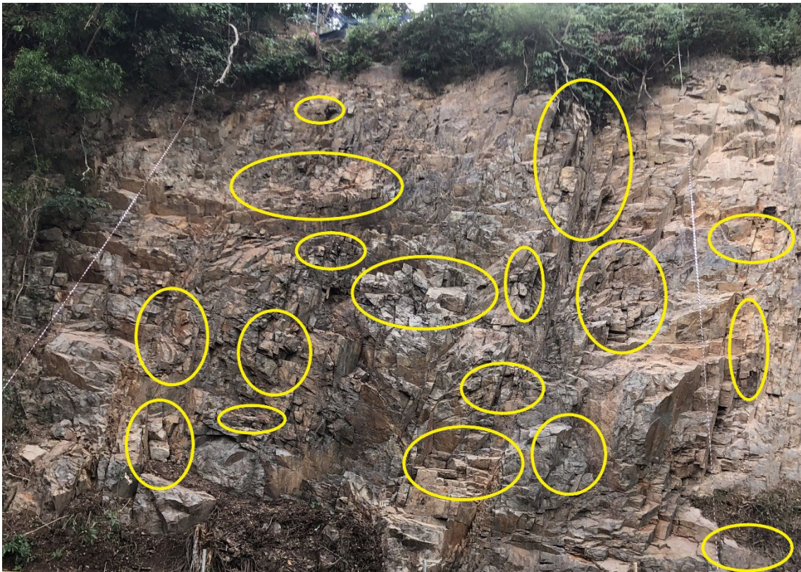
FIG 6 – Area of focus for scaling work.
