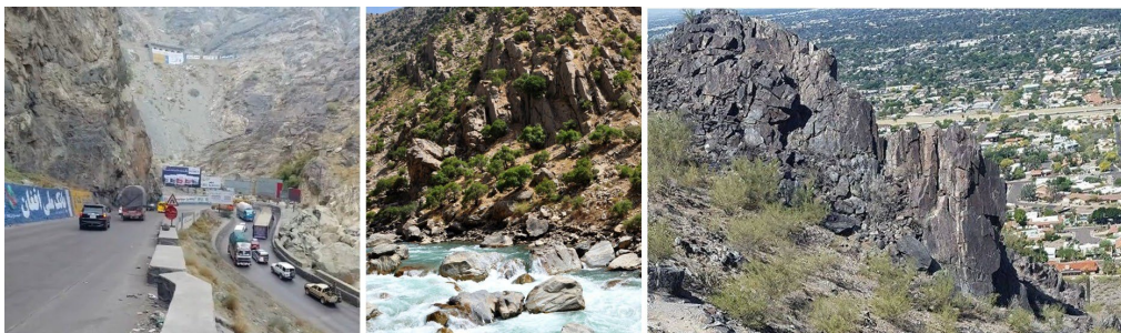
FIG 6 – Slope failures belonging to Category III involving columnar toppling.
