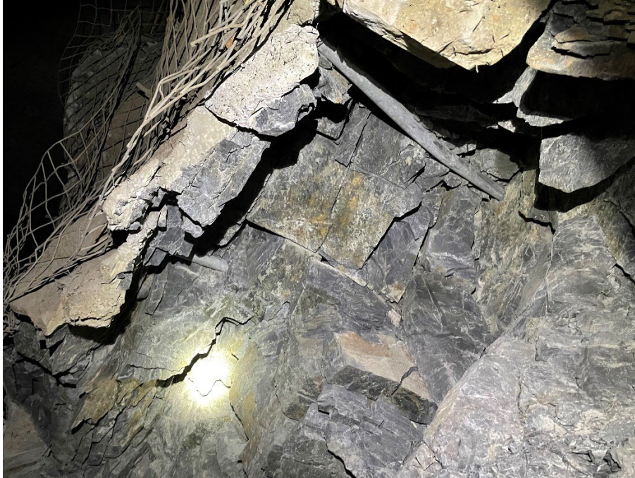
FIG 4 – A failure site with an overhang.
