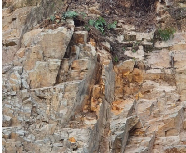
After scaling work
