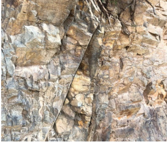
Before scaling work
