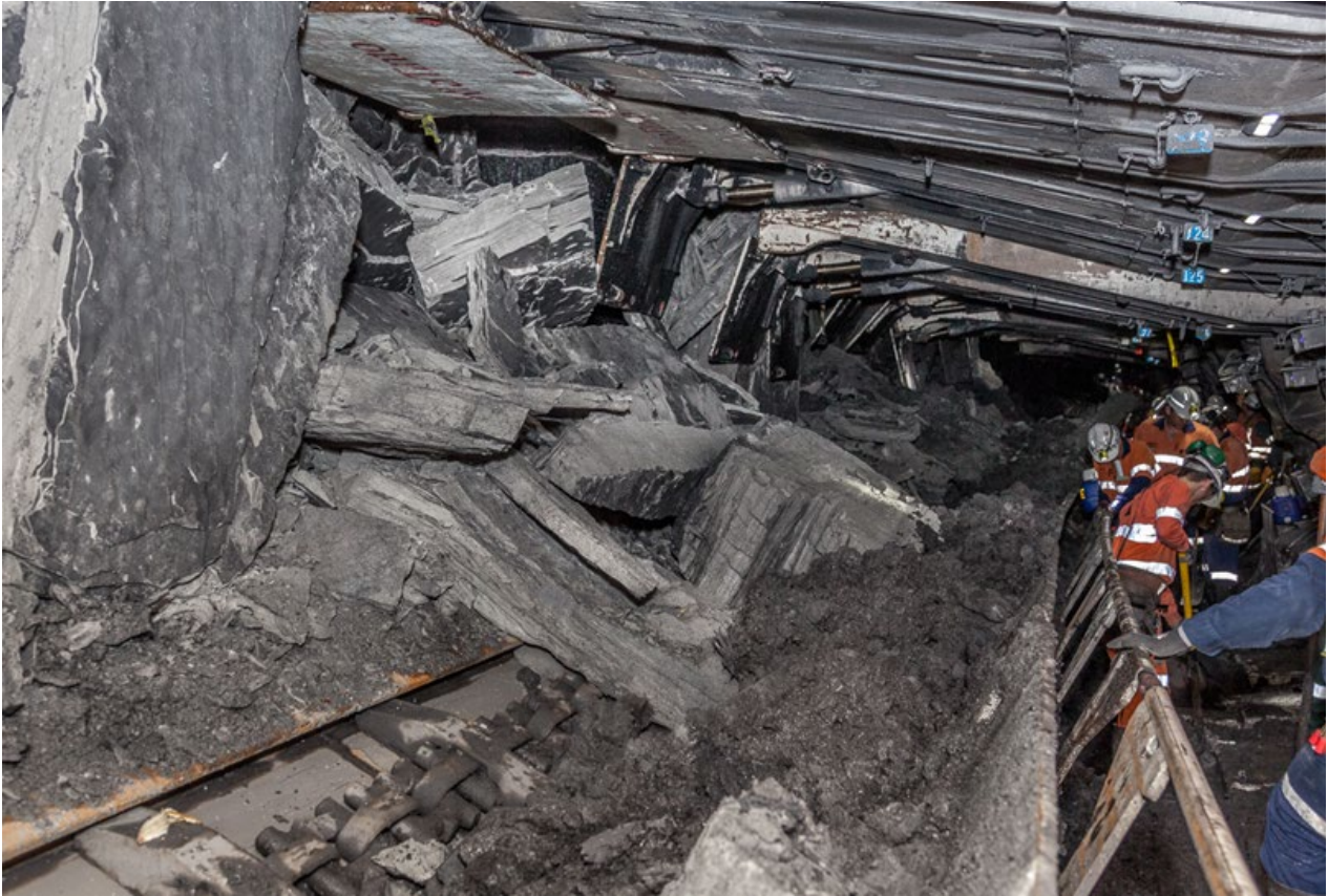
FIG 1 – Roof failure at the longwall face following severe floor heave event.
