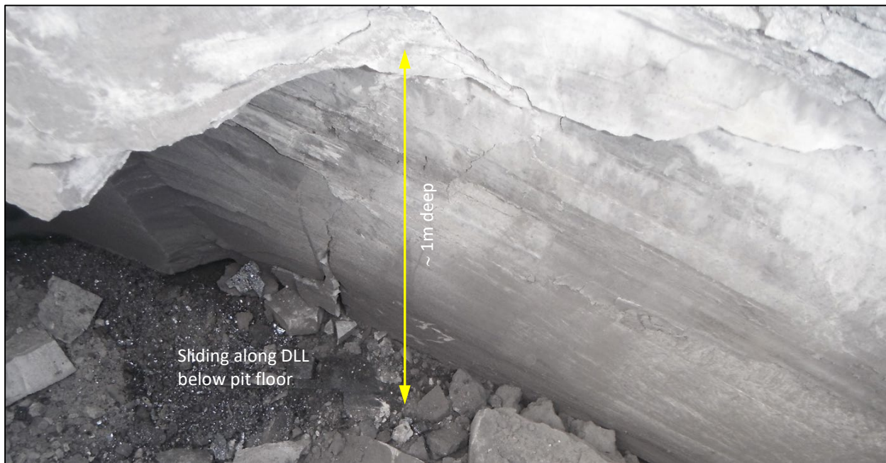
FIG 10 – Shear below floor observed from a floor disruption blasting induced dragline lowwall failure in one of the northern pits.
