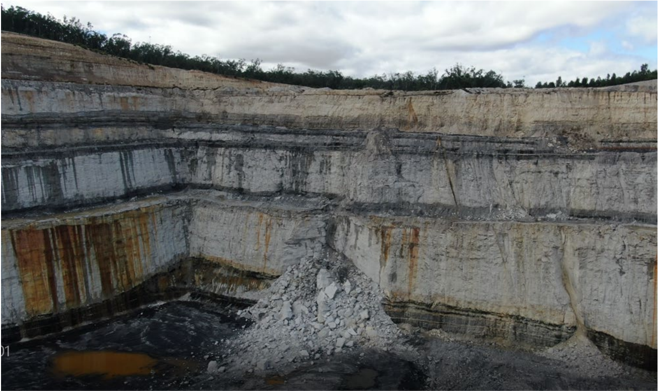
FIG 3 – Highwall rock mass failure.
