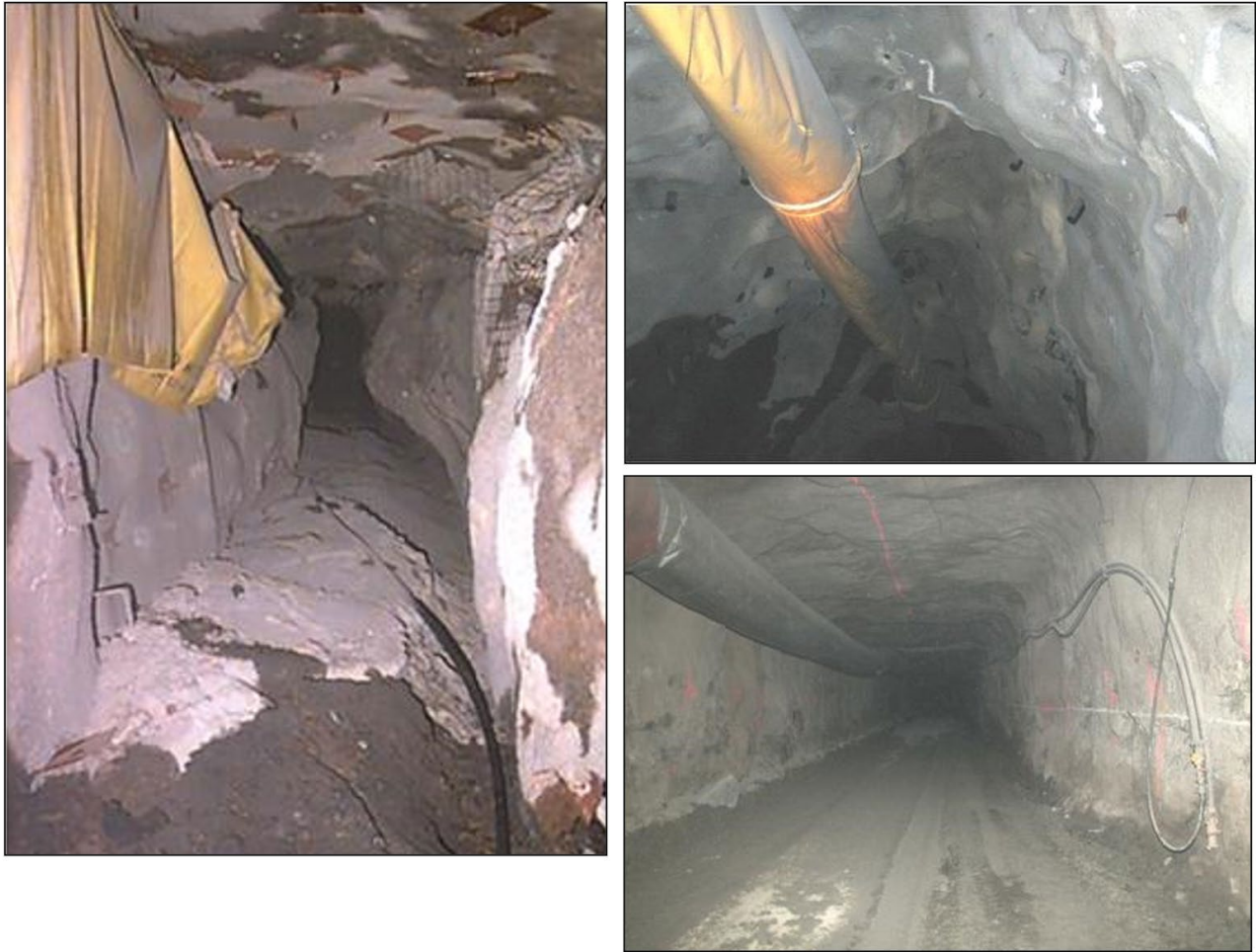
FIG 2 – Various ground conditions and rock mass response in SLC mines. Clockwise from the left, squeezing conditions at the Perseverance mine (after Struthers et al, 2000), jointed rock mass prone to wedge failure at Stobie (after Power and Just, 2008) and favourable rock mass conditions without major ground control problems at the Ridgeway SLC (after Power and Just, 2008).
