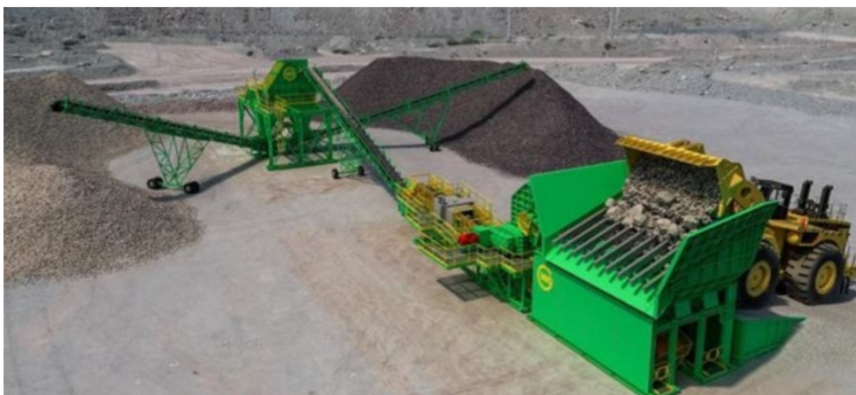
FIG 5 – GEOSCAN analyser in a copper ore bulk sorting plant at El Soldado, Chile (source: Hillyer, 2019).
