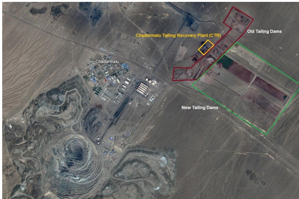
FIG 1 – Location of old and new tailings dams to accumulate wet tailings from the Chadormalu iron ore processing lines.
