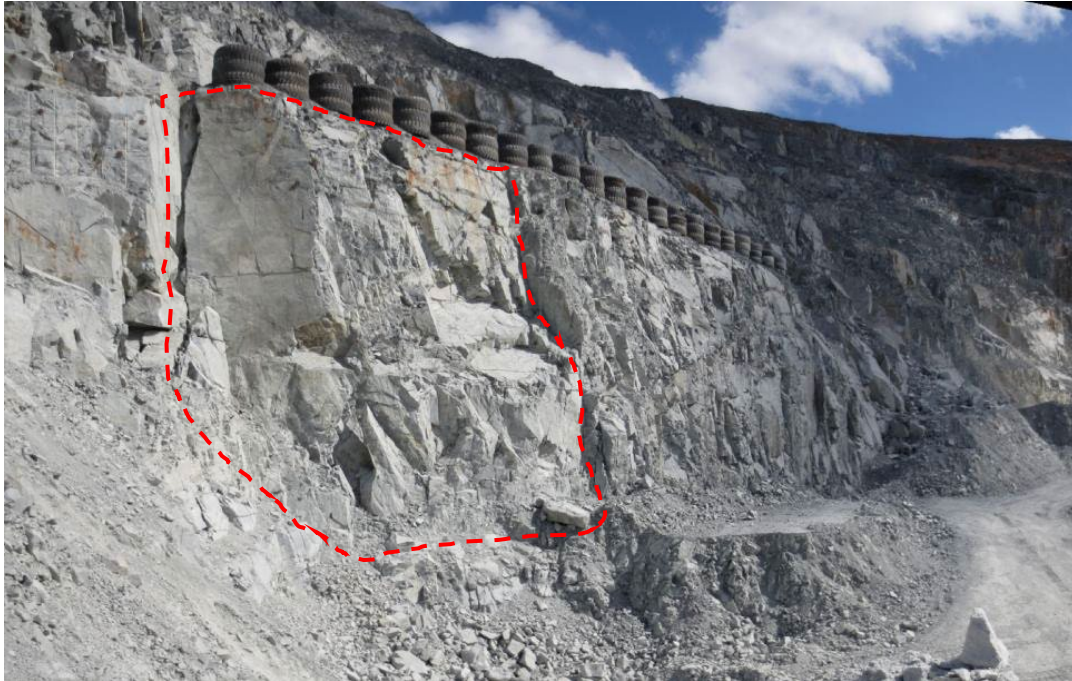
FIG 5 – Photo showing the block and the controlling structures.
