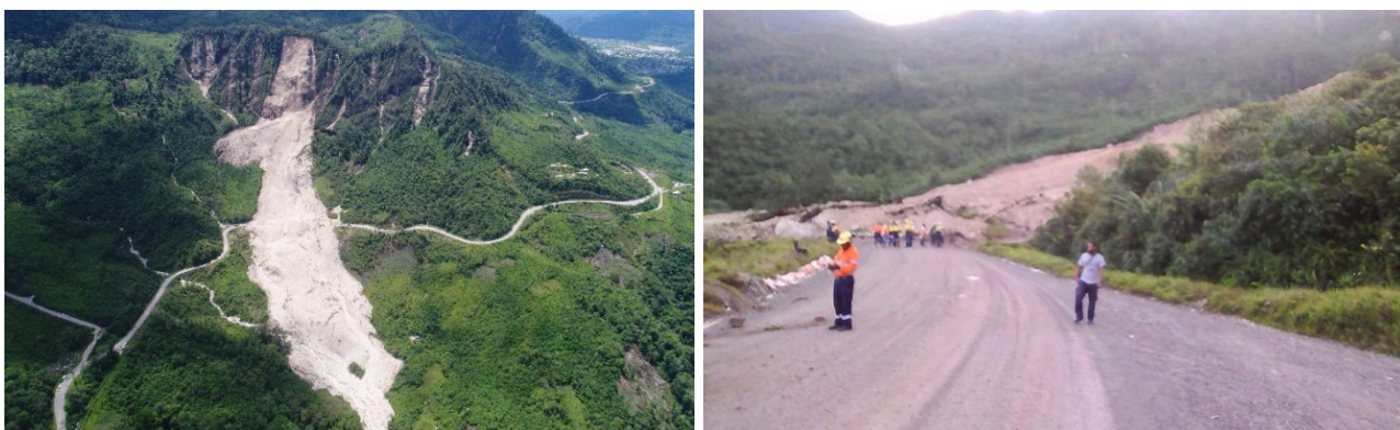
FIG 1 – 26 Feb 2018 Earthquake in PNG resulting in failure of natural slopes, blocking mine access road: (left) aerial view; and (right) debris pile at access road.
