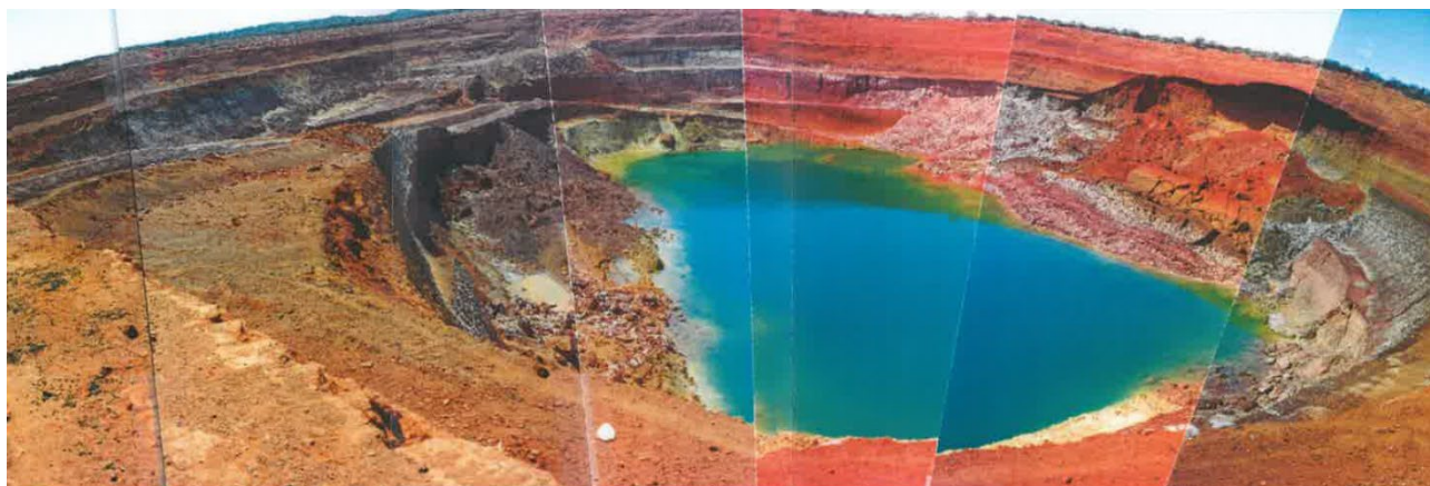
FIG 6 – Panoramic view of the pit circa 2002 showing the extent of failure.
