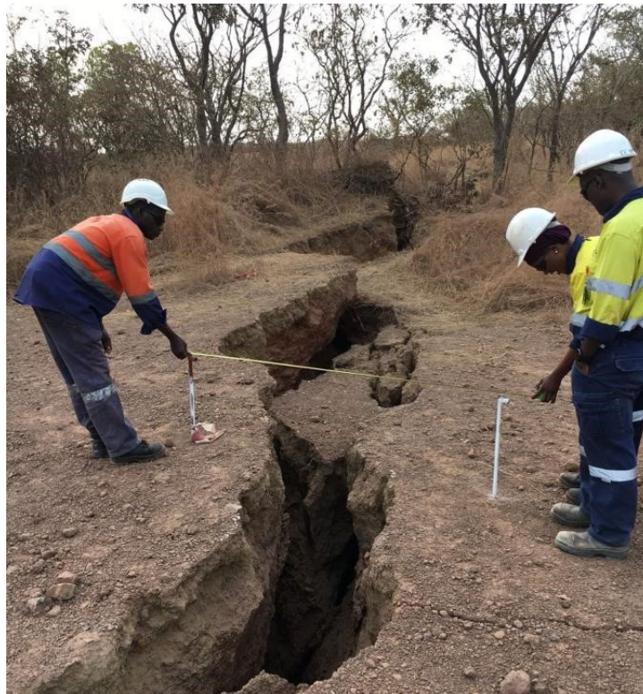
FIG 9 – Personnel conducting crack pin measurements in December 2019.
