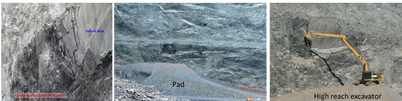
FIG 10 – Long reach excavator remediation.
