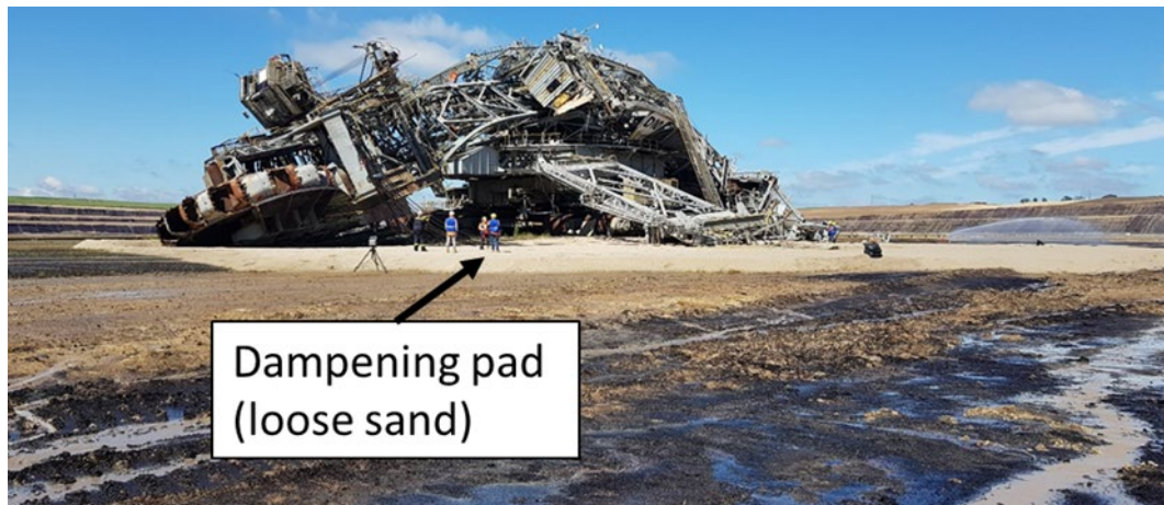
FIG 17 – Post-demolition inspection – Dredger D11.
