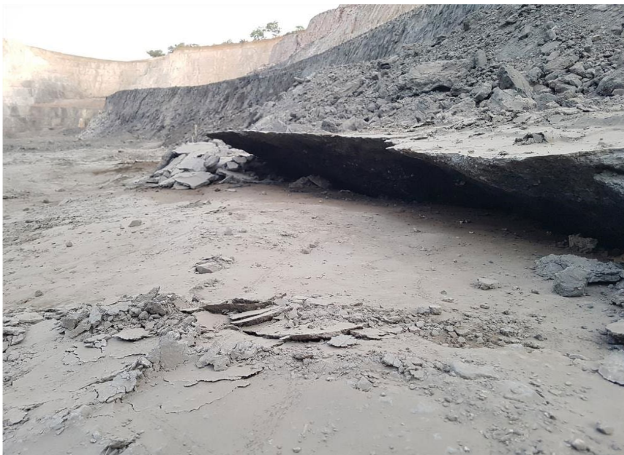
FIG 18 – Floor heave in Namakan pit.
