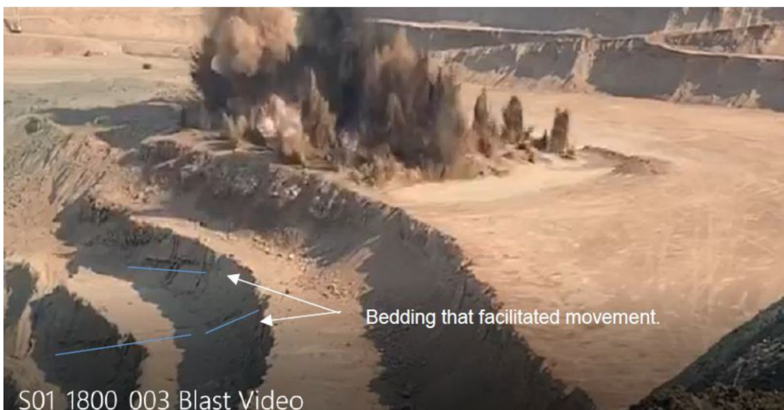
FIG 4 – Blast-induced movement on structures in adjacent benches.
