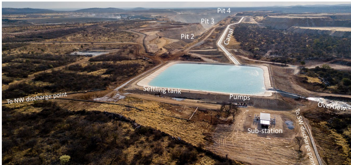
FIG 5 – Key dewatering distribution infrastructure at Tschudi (from Sarma, 2018).
