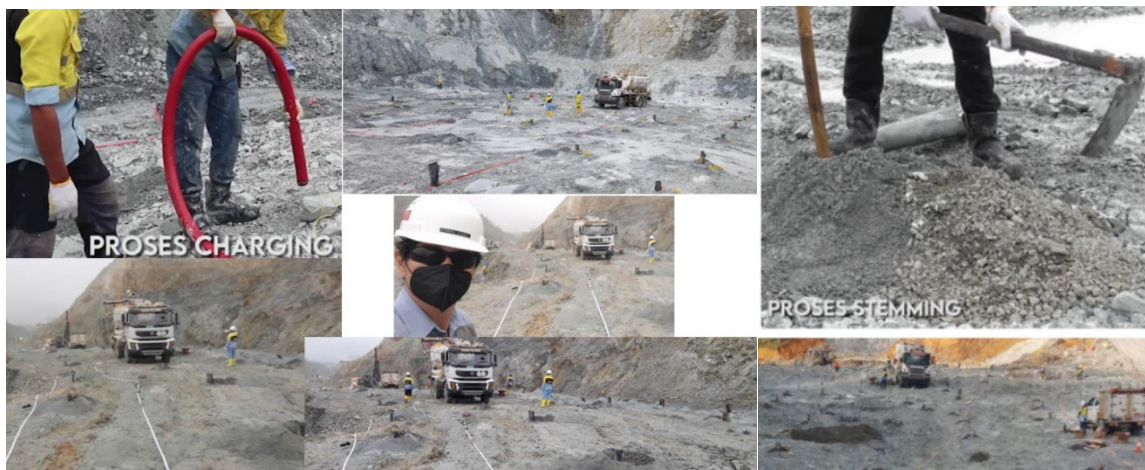
FIG 9 – Charging explosives and stemming process.
