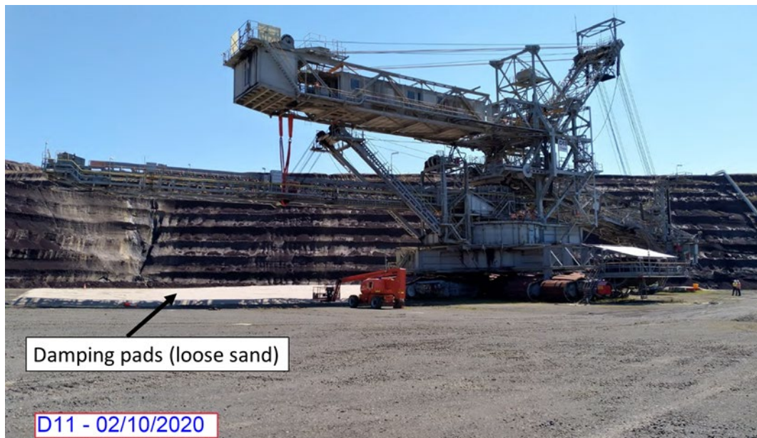
FIG 16 – Pre-demolition inspection – Dredger D11.
